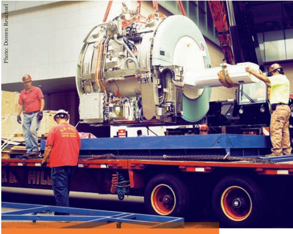
The 13-ton MRI scanner is hoisted by a crane outside the Martinos Imaging Center.
